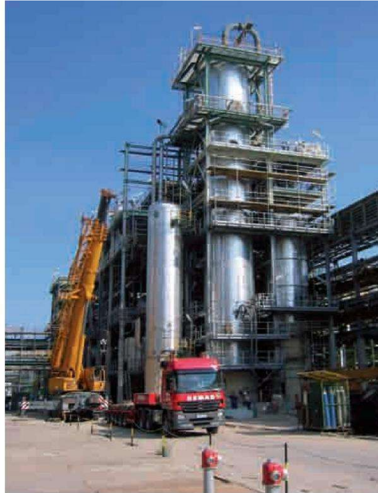
Erection of oxychlorination reactor BorsodChem Rt., Hungary
